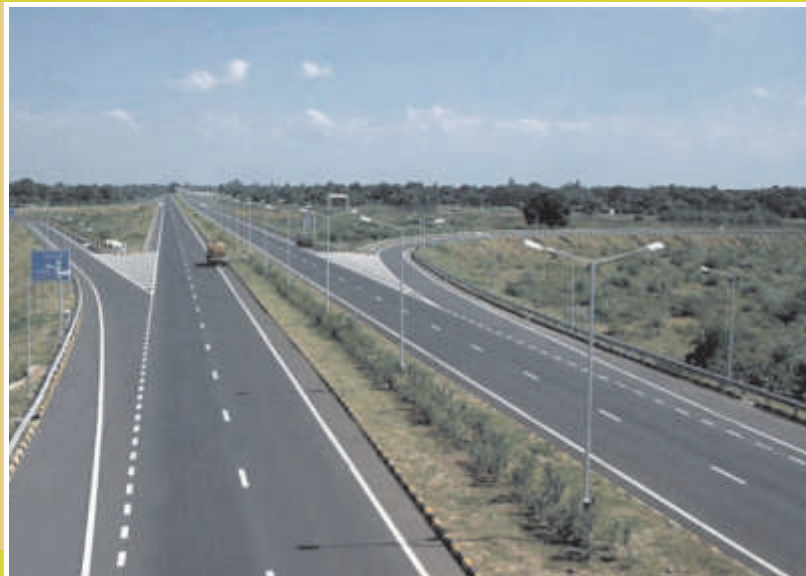
4 Lane & 6 Lane Highway (Dhar, Ujjain, Ratlam, Neemuch, Raj., Guj., Link High-way)
